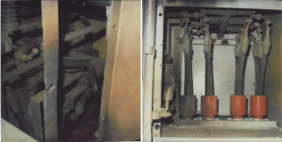
Fig. 5. Photographs: a) view into the exciter cabinet, in the foreground location where the screw loosened and b) view into the cabinet
