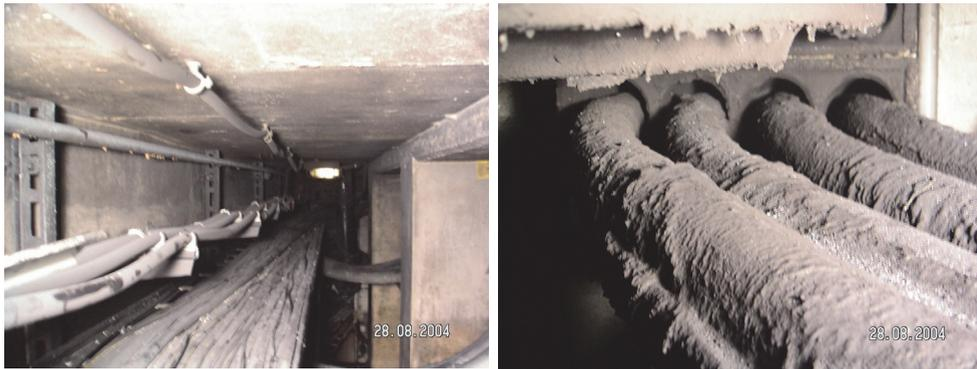
Fig. 4. Cables with protection by intumescent coating; left: photo of the cable channel, right: photo of the coating
