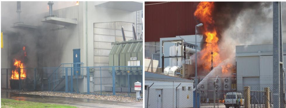
Fig. 8. Flame and smoke occurring at the generator transformer; the photo on the right hand shows the fire extinguishing activities
