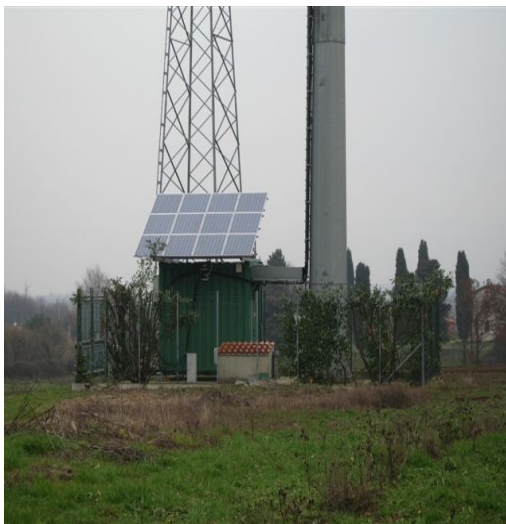
Fig. 11. Photovoltaic system installed on the BTS infrastructure (Vodafone)
