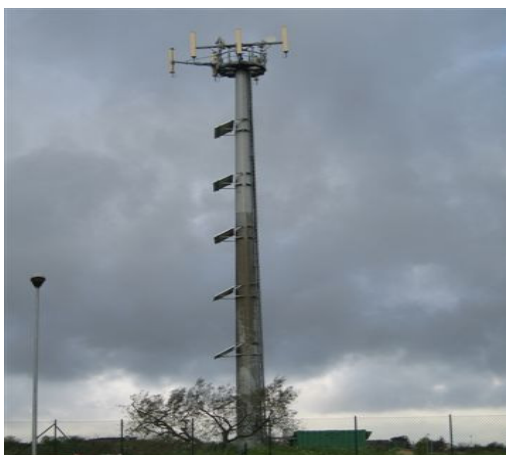
Fig. 12. Photovoltaic system installed on the BTS infrastructure (Vodafone)
