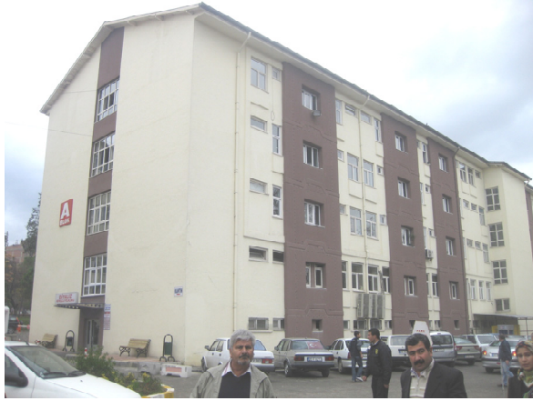
Fig. 8. An external shear wall strengthened building
