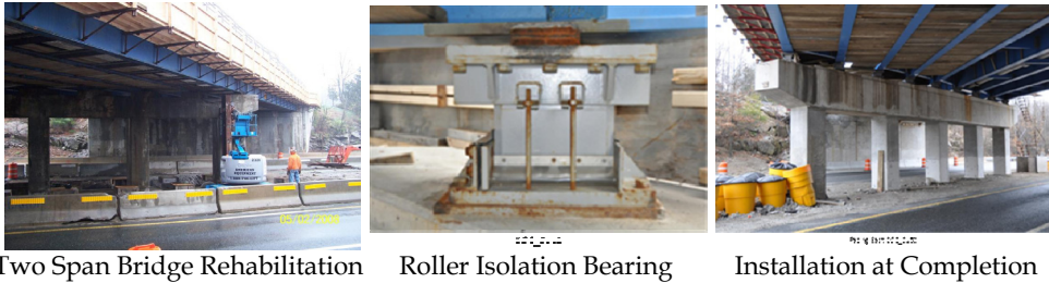
Fig. 5.3. Bridge Rehabilitation in Rhode Island
