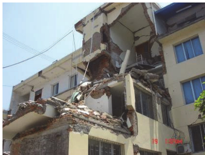
Fig. 3. Partial collapse of stair part
