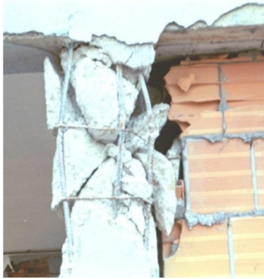
Fig. 9. Shear failure of column (Italia 2002)
