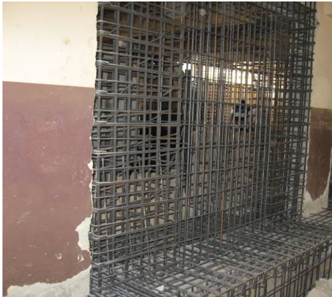
Fig. 3. Infill wall application in an RC building
